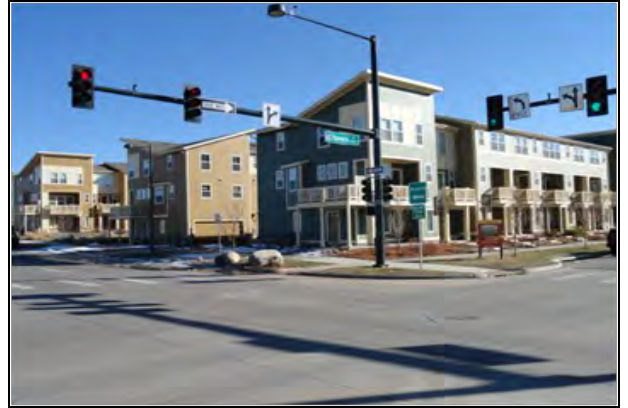
29th Drive Row Homes Denver, Colorado
